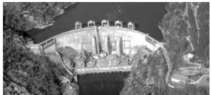
The Smith Mountain Project is a 636-megawatt pumped storage hydroelectric facility.
